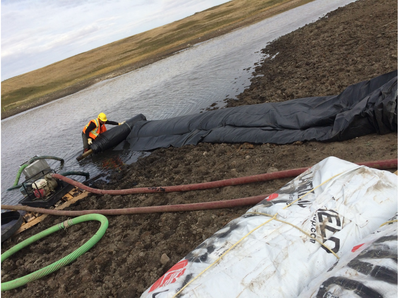
Aquadam being constructed.
